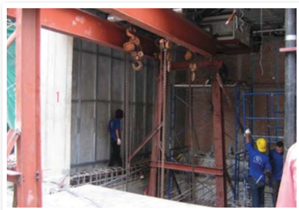
Figure 1: The installation site for cyclotron.
